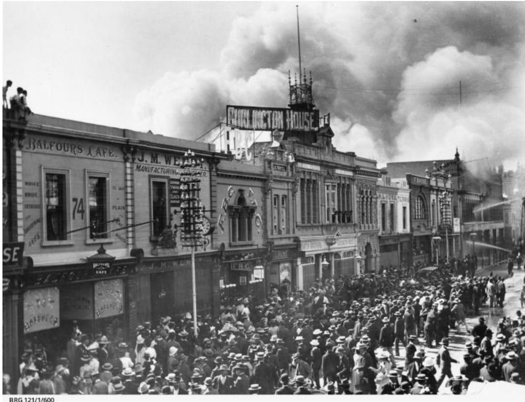
State Library of South Australia - Street scene during John Martin's fire [BRG 121/1/600], View looking east along Rundle Street towards the fire in the John Martin's store on April 6 (Easter Saturday) 1901. 70,000 pounds worth of damage was done and one side of the building was reduced to ruins. Firefighters are aiming hoses at the building while smoke billows across the sky. A large crowd of onlookers fills the street. A range of shop fronts can be seen including the Balfours Cafe, J.M. Wendt, F.B.C. and Burlington House. [From scrapbook 92]. Copyright restrictions may apply. David Jones, Botanicca, Building 2, 572 Swan St, Richmond VIC 3121. Copies may be made for research or study. Publication only with written permission from David Jones. All use must acknowledge David Jones Ltd. 1901. Part of John Martin Collection.
