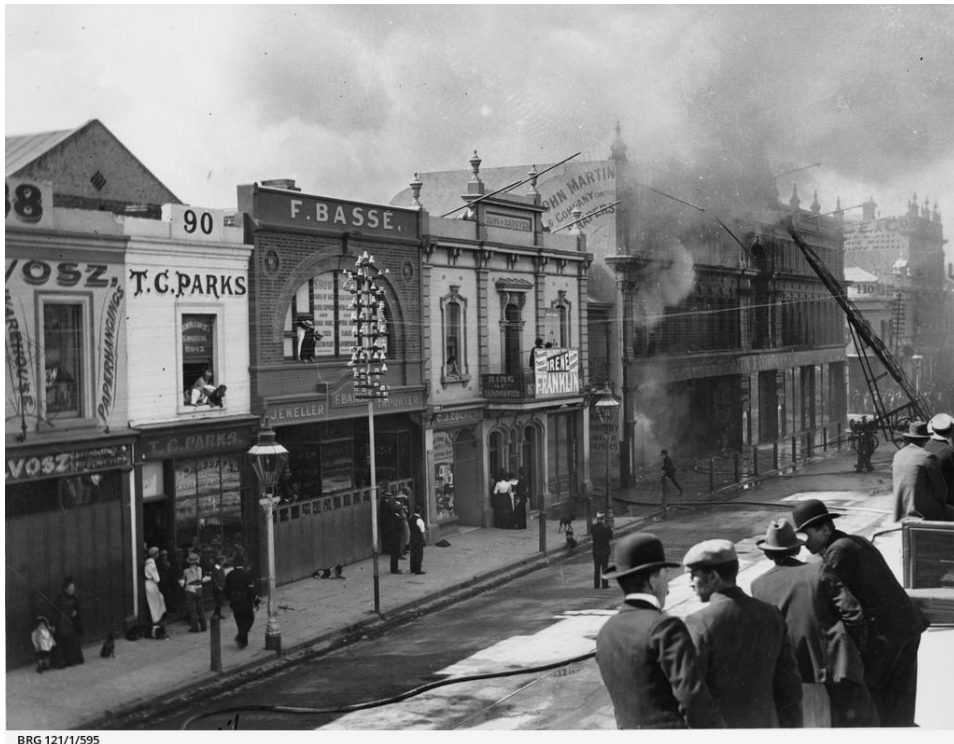
State Library of South Australia - Fire at John Martin's store [BRG 121/1/595], View looking north-east across Rundle Street at the fire in John Martin's store on 6 April 1901 (Easter Saturday). Smoke is billowing from the top of the building and a firemen's ladder is being used, while groups of bystanders look on. A number of other shop fronts are in view, including T.C. Parks, F. Basse and the King of Hanover Hotel. [From scrapbook 92]. Copyright restrictions may apply. David Jones, Botanicca, Building 2, 572 Swan St, Richmond VIC 3121. Copies may be made for research or study. Publication only with written permission from David Jones. All use must acknowledge David Jones Ltd. 1901. Part of John Martin Collection.
